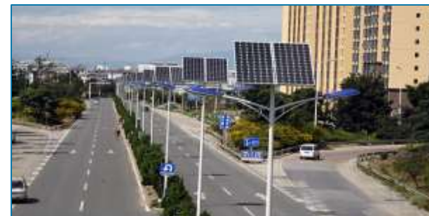
Solar streetlights in China (10kW shown)
