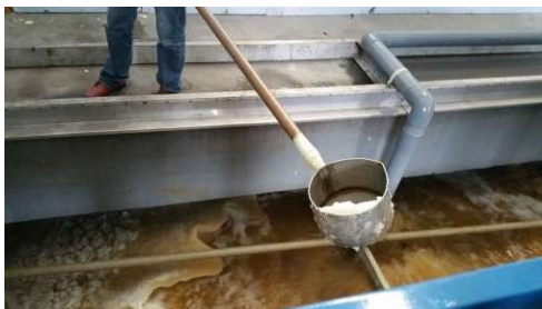
Dynamic ice storage in DC of Chengdu (In operation)
