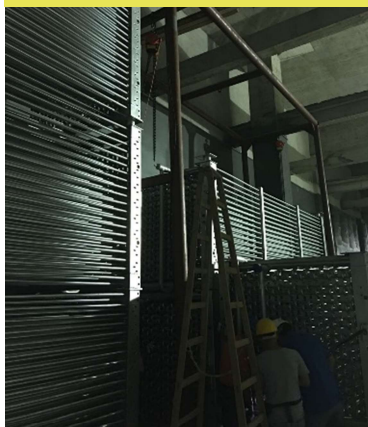
Ice storage coils in DC of Shenzhen (Construction stage)
