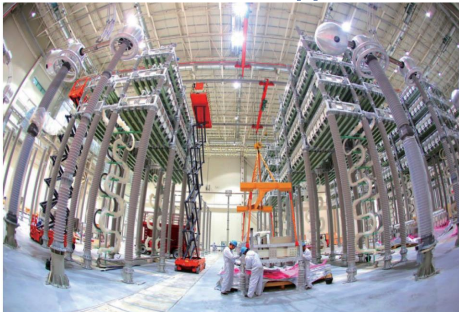
Figure 2 Zhangbei Flexible DC Power Grid Demonstration Project and Flexible DC Transmission Equipment (II)
